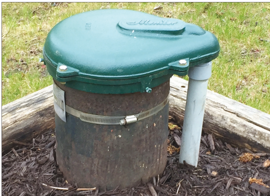
Photo above: well in good condition.
